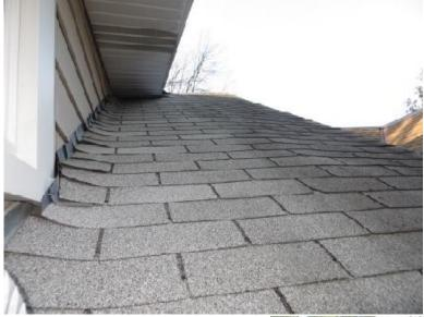
7. ☐ Valleys: Preformed metal Valleys are rusted. Roof patch at area of former chimney penetration has fiberglass 3 tab shingle as upper portion of valley and is incorrect installation.
